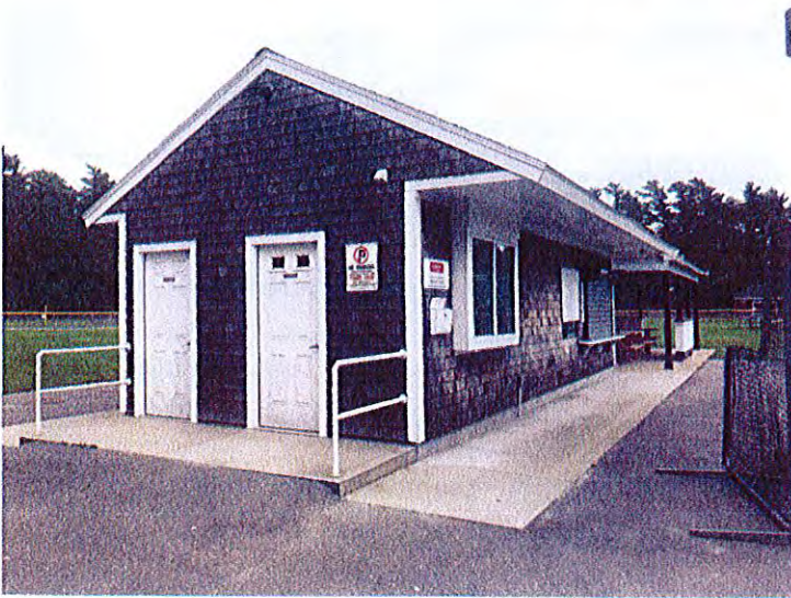
ADA Bathroom and Snack Shack
